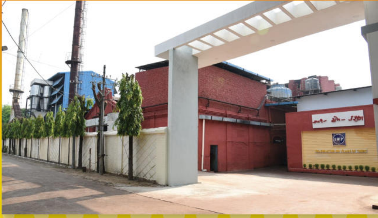
Plant at IZZATNAGAR, Barielly
