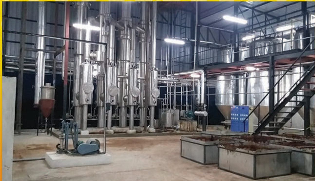
Plant at Jammu & Kashmir under Installation
